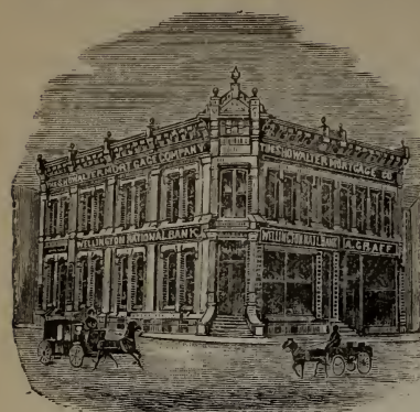
Western Offices, Wellington, Kansas.
